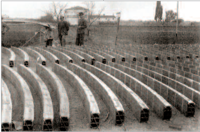
Above Construction elements for the covering of the new warehouses, before the installation (1945).
