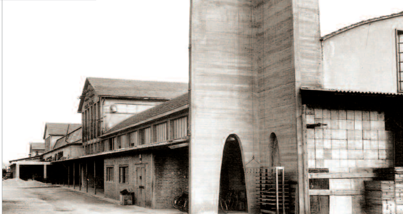
Next The fire-fighting piezo metric tank, which became almost an ideal "campanile" (bell tower), symbol of the company (1945).
