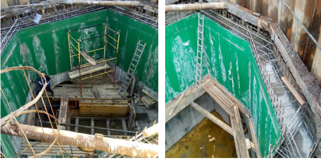
RESTORATION OF THE SEWAGE COLLECTOR DISCHARGE CHAMBER
