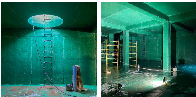
CLEAN WATER RESERVOIRS FACED WITH DRINKING QUALITY LINING SHEET.
