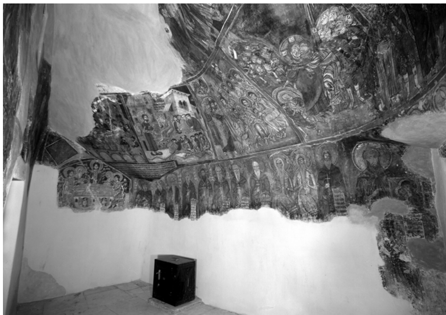
10. Naos, looking southwest (photo: Ann Wharton, courtesy of Dumbarton Oaks)
