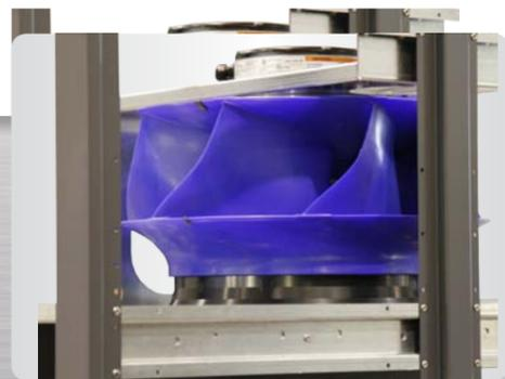
EC fans (standard for the entire range) vary the airflow to match heat load requirements. This translates into a more efficient fan energy use and, as a result, a lower PUE for the system.
